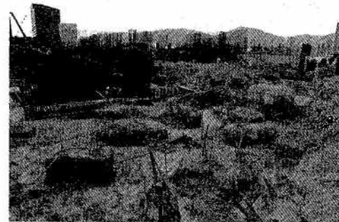
Fig 2.3 1600mm diameter hand dug caissons adopted where depth to bedrock was less than 5–6m
