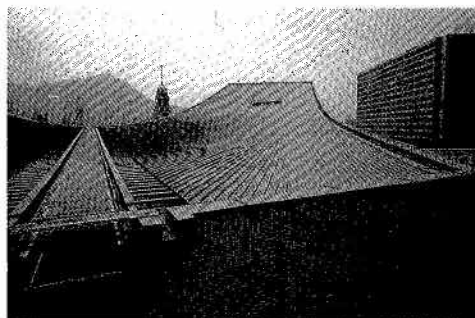
Fig. 4.13 Sweeping surface of completed Cultural Centre roof
