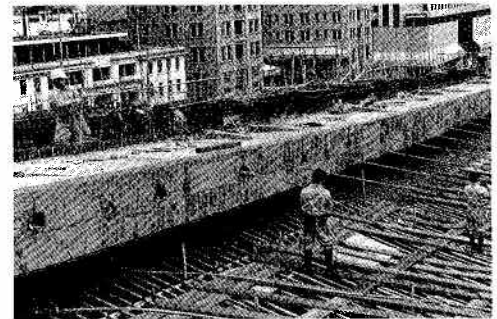
Fig. 4.5 Work on cable erection
