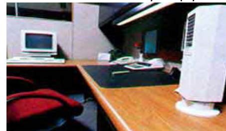
Desktop air supply pedestals
