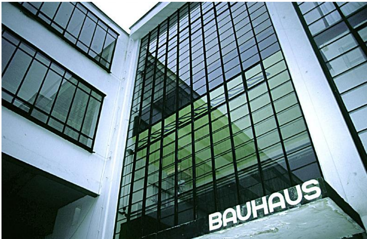
Bauhaus, glass façade, Walter Gropius
