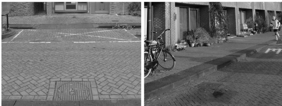
Services man-hole cover embedded in road at Borneo-Sporenburg. 22
