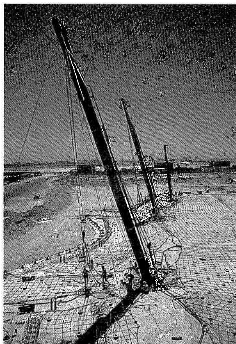
Fig 6.6 Preparations for lifting cable net
