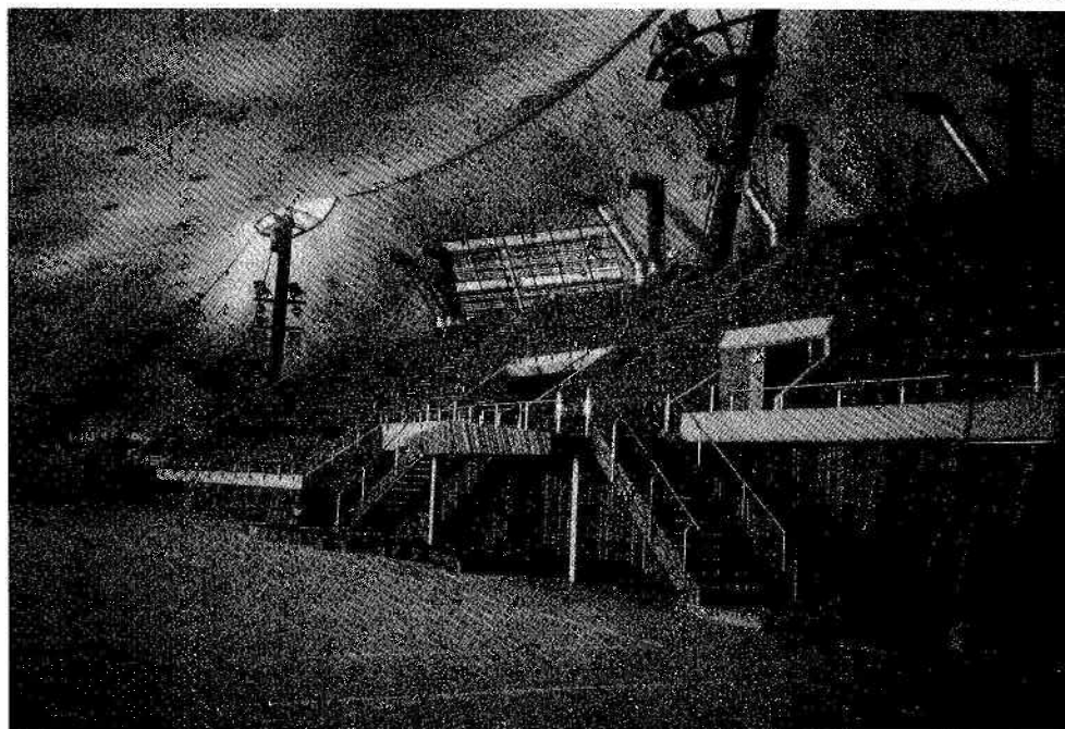
Fig 6.16 View of finished interior
