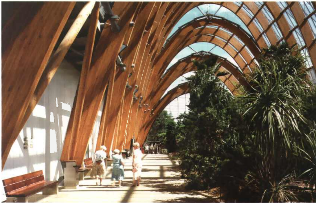
The arched glulam structure of the Sheffield Winter Garden creates a dramatic interior.
