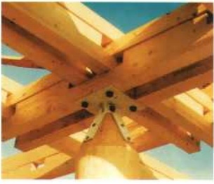
The hall roof at West Totton school is supported by cylindrical glulam columns; they taper at the head to support a grillage of glulam beams.
