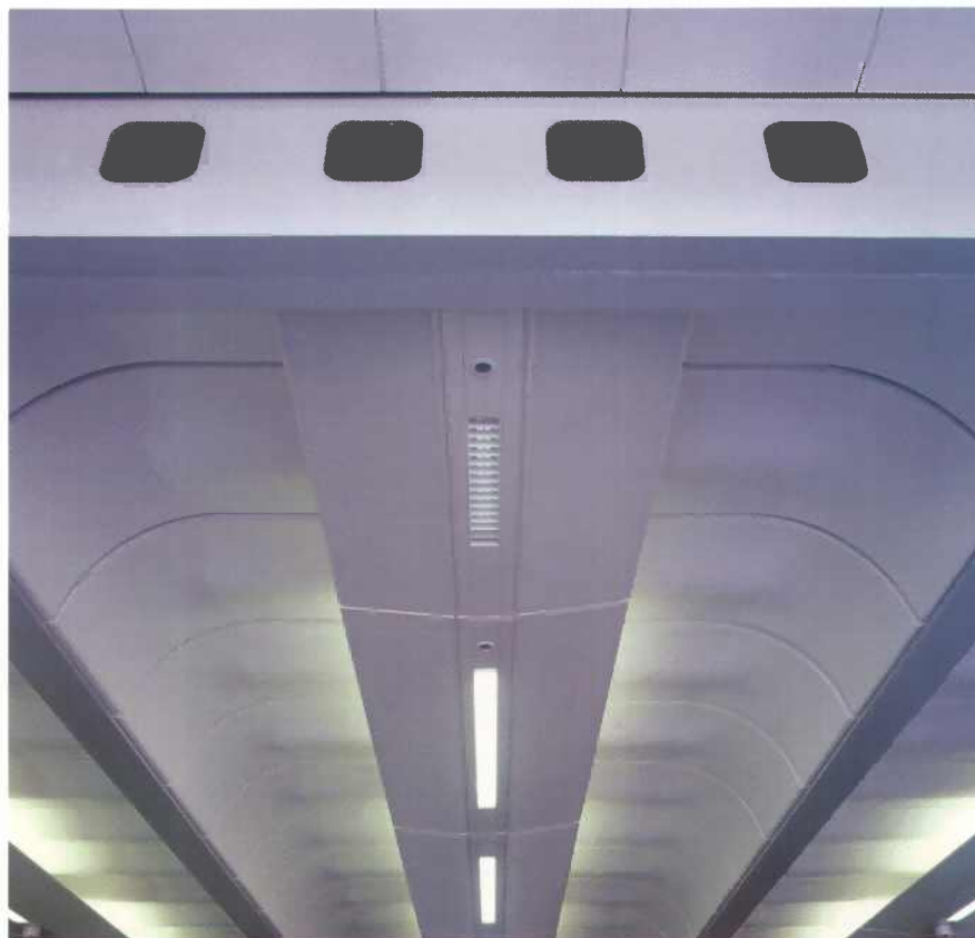
The concrete floors of the Wessex Water headquarters in Bath contain recycled aggregate.
