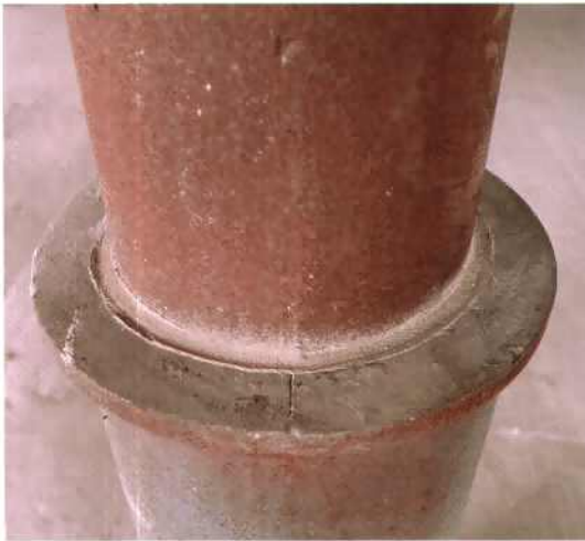
Column with strapping
