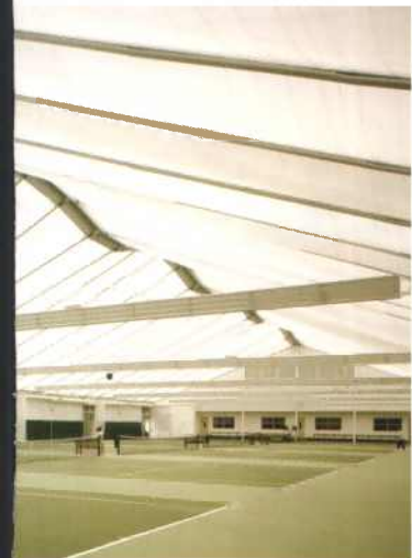
The internal view of Hampshire Health and Tennis Centre shows the large, well-lit space created by the ETFE roof structure.
