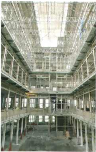
The mill interior had a delapidated atrium.
