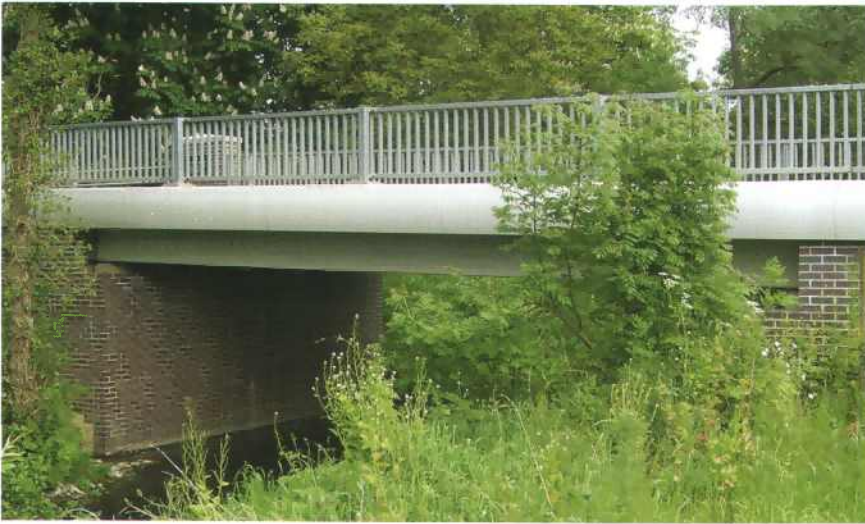
The west mill bridge in Oxfordshire, opened in October 2002, is the first public highway bridge in Europe to be built from advanced composite materials. Its structural performance is being continuously monitored by a fibre-optic system with Bragg-grating sensors, data from which are to be collected remotely for analysis. The bridge, constructed from a hybrid glass/carbon composite material, was developed as an EU project led by Mouchel Parkman
