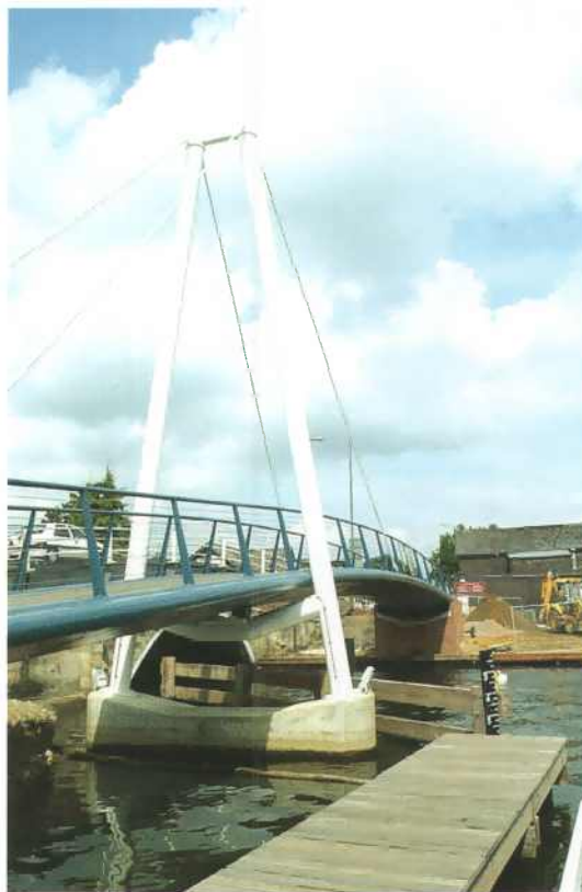
The soffit of a pedestrian footbridge at Wroxham is clad with 2m-wide GRP panels which provide a crisp finish and contain services.
