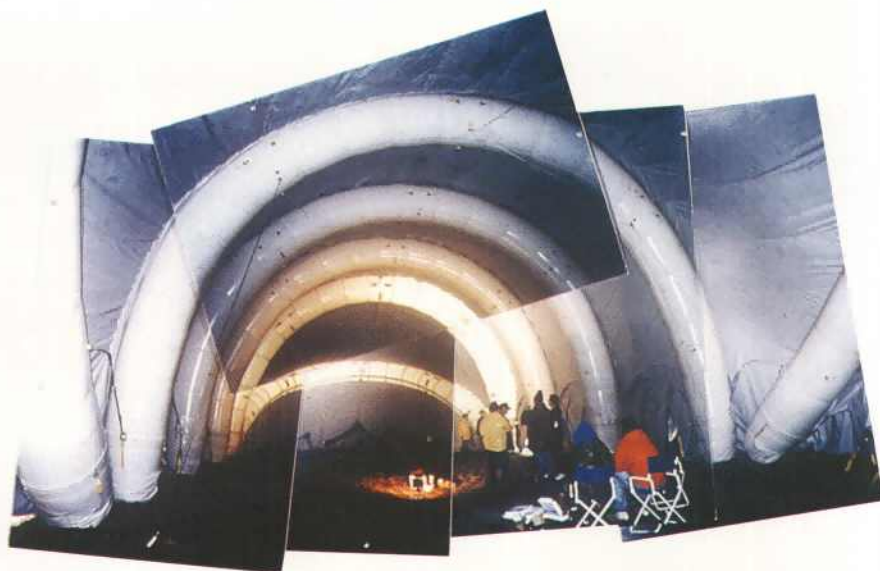
Internal view of TME, showing bulky nature of polyester air beams.
