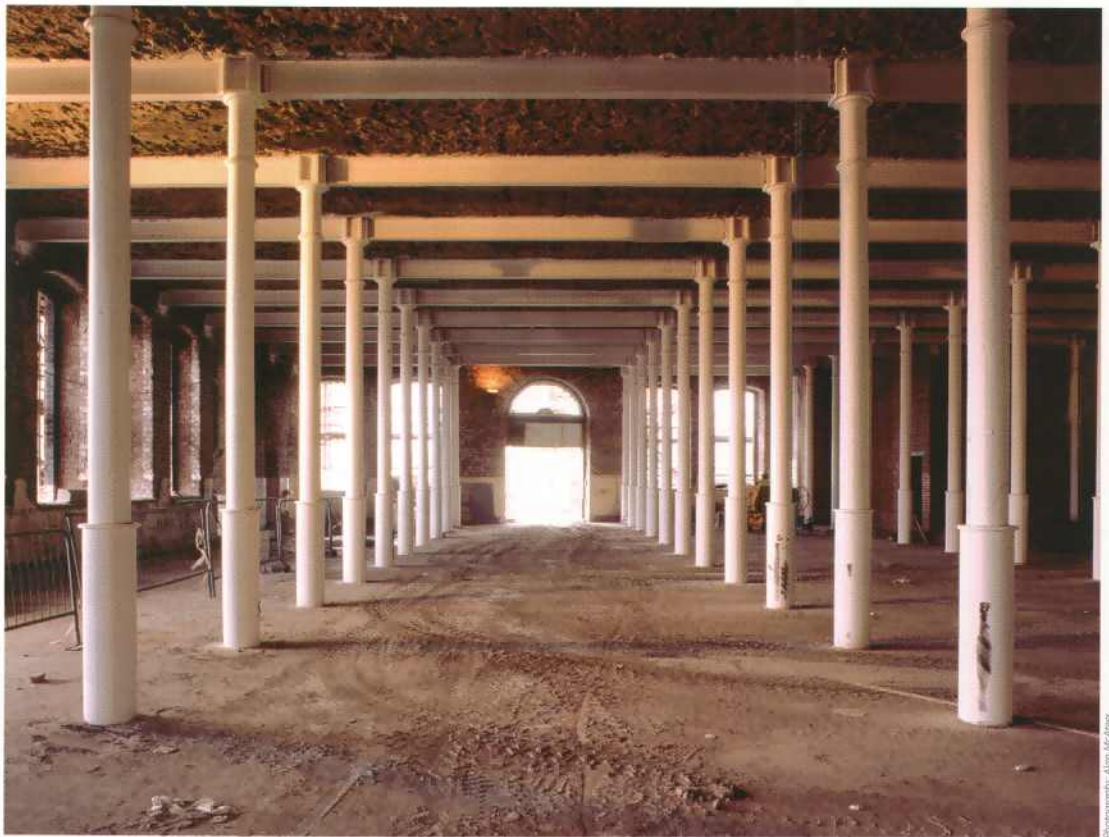
The saddle box and cast iron columns
