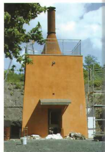
A view of the experimental lime kiln (ELK) at Paisley University.
