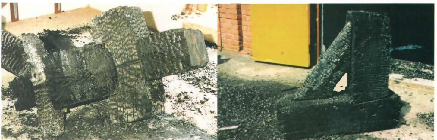
Successful fire tests on untreated oak, jointed with traditional details for the Globe Theatre, London, led to an increased respect for traditional craft skills.
