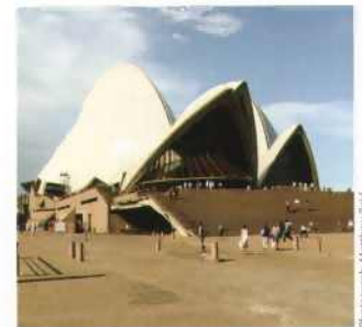
The concrete shell structures of the Sydney Opera House were bonded together by means of epoxy resin adhesives.
