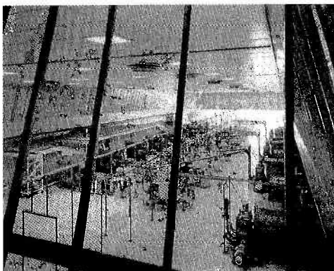
Fig 5.5 Main hall seen from 1st floor visitors' gallery
