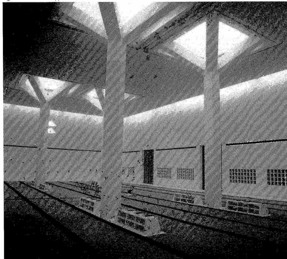
Fig 11.2 Internal support columns to roof
