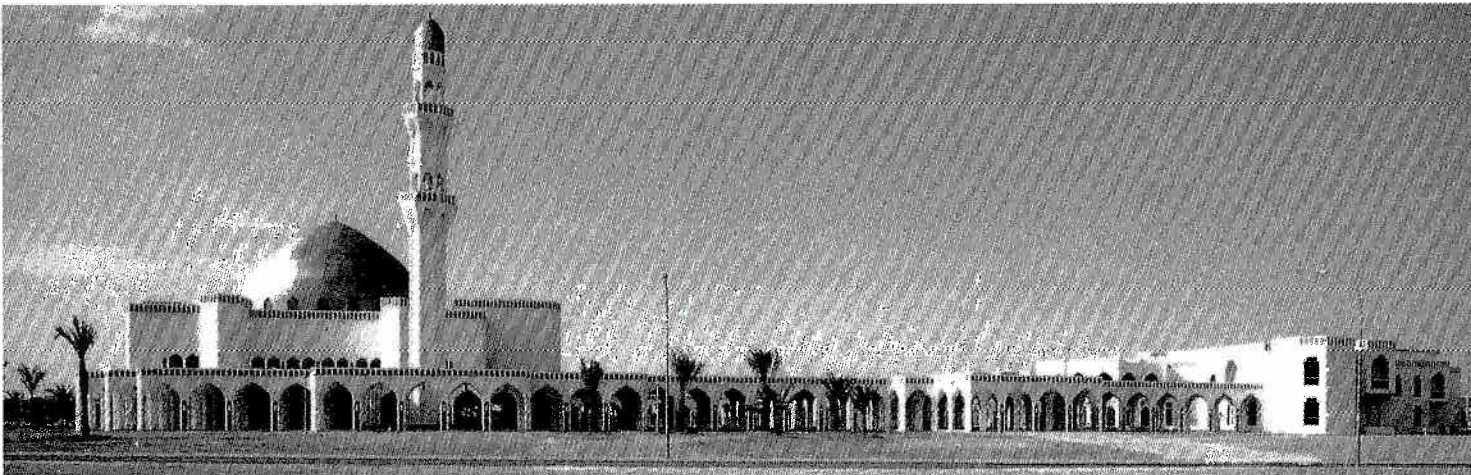
Fig 5.2 The completed project, viewed from the north
