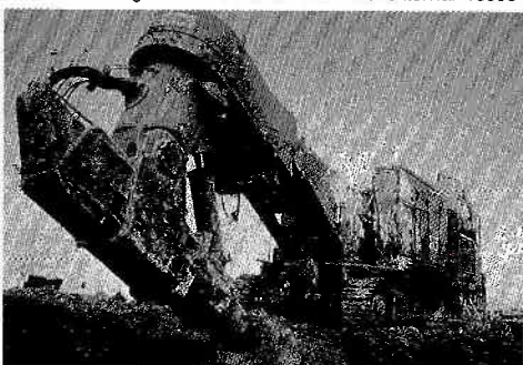
Fig 12.4 Rock breaking equipment used on site
