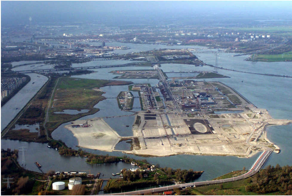
12. IJburg Under Construction
