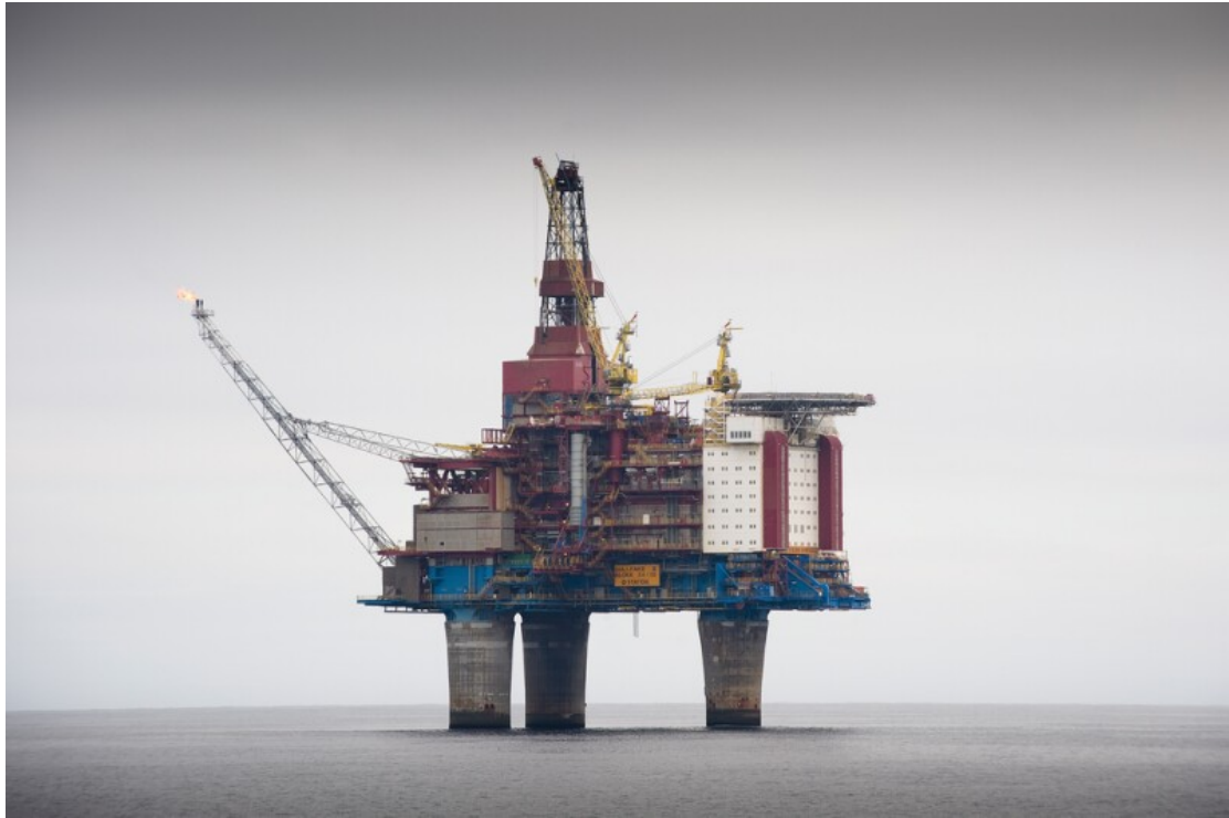
2. A concrete production platform in the North Sea
