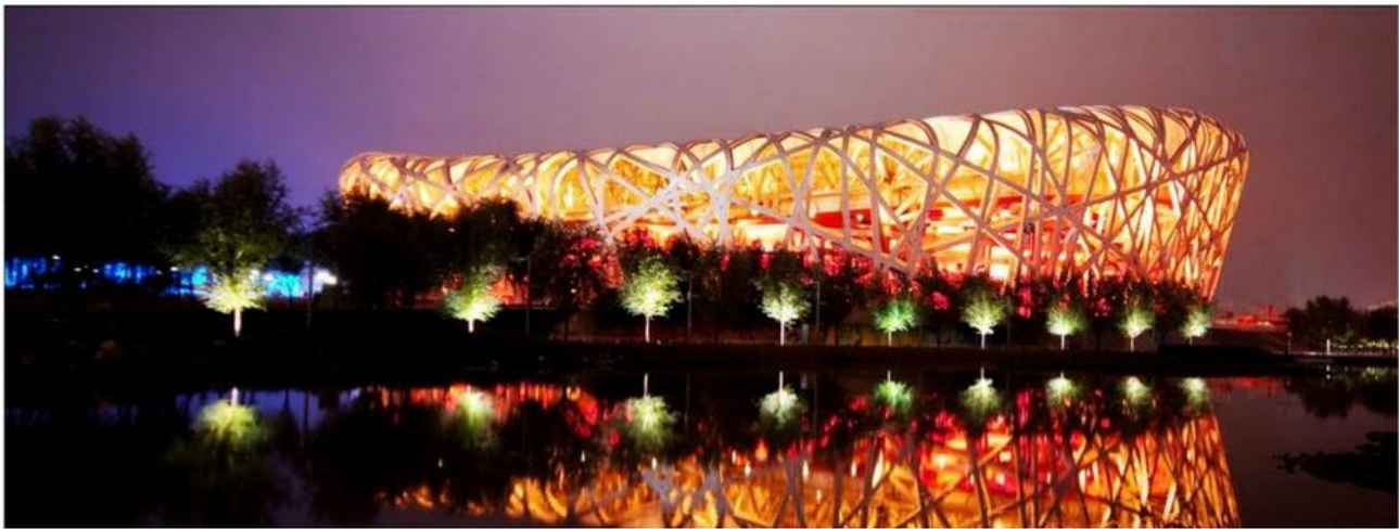
The night view of the stadium(google)
