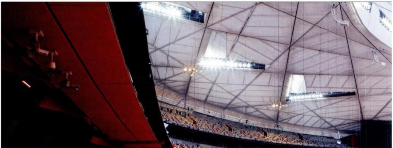
Single-layer ETFE membranes stretched between the steelwork sections protects the spectators from wind and rain. (google)
