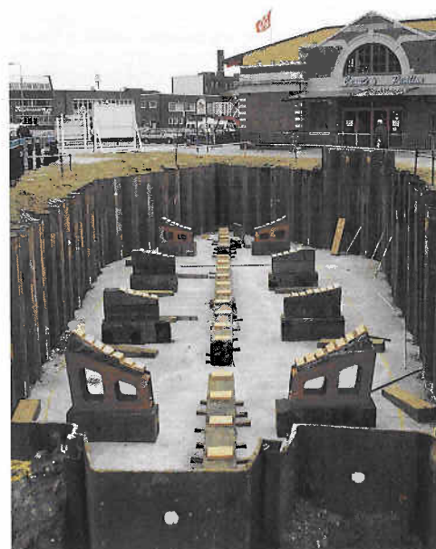
Fig 2.2 Purpose-built dock awaiting transfer of lightship
