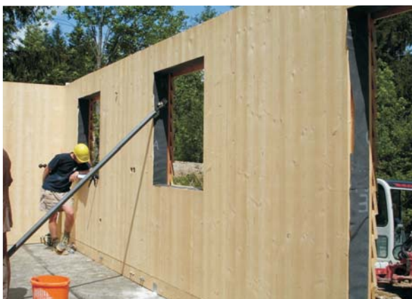
prefabricated BBS-wall including electrical services, insulation and facade
