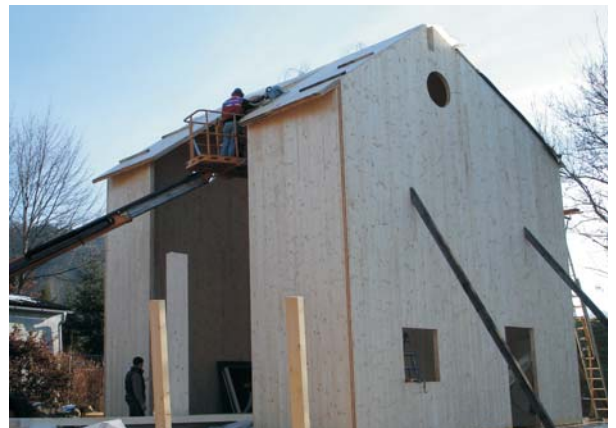
BBS multi storey wall
