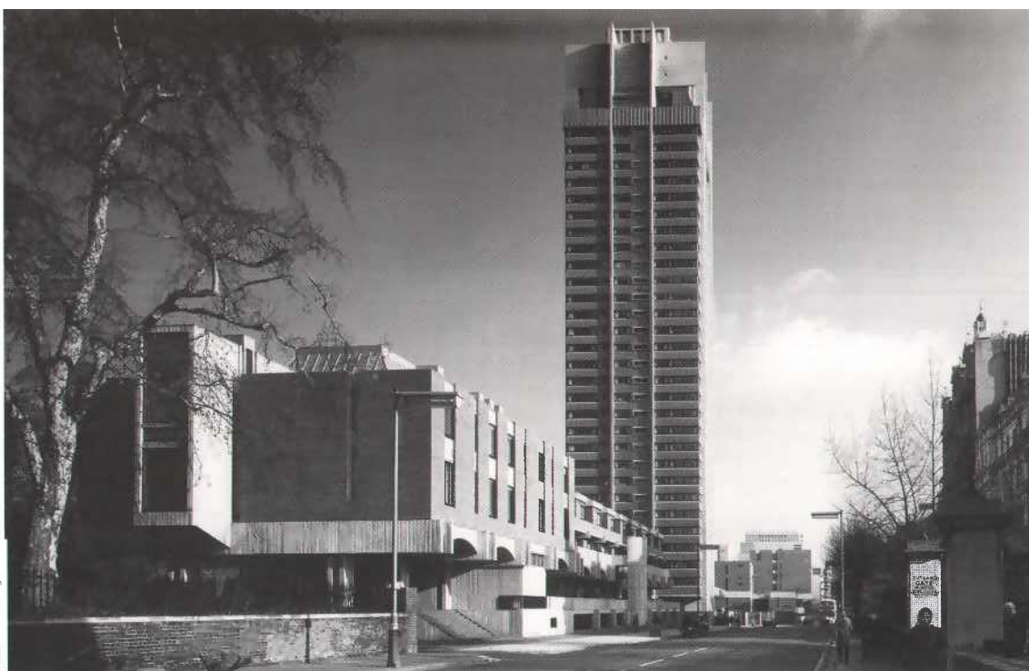
Knightsbridge Barracks Engr: OAP Structures 3 Arch: Sir Basil Spence Partnership Date: 1960-70
