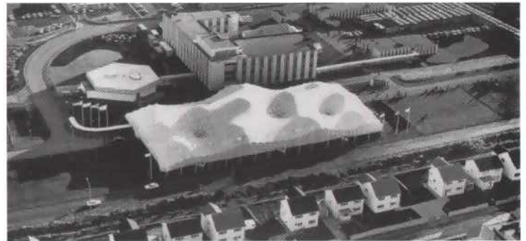
Dyce tent, Forties Field Engr: OAP Arch: Design Research Unit, Frei Otto Date: 1975
