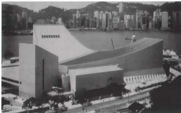
Tsim Sha Tsui Cultural Centre, Hong Kong Engr: Buro Happold Arch: Hong Kong Public Works Dept. Architects Date: 1981-89
