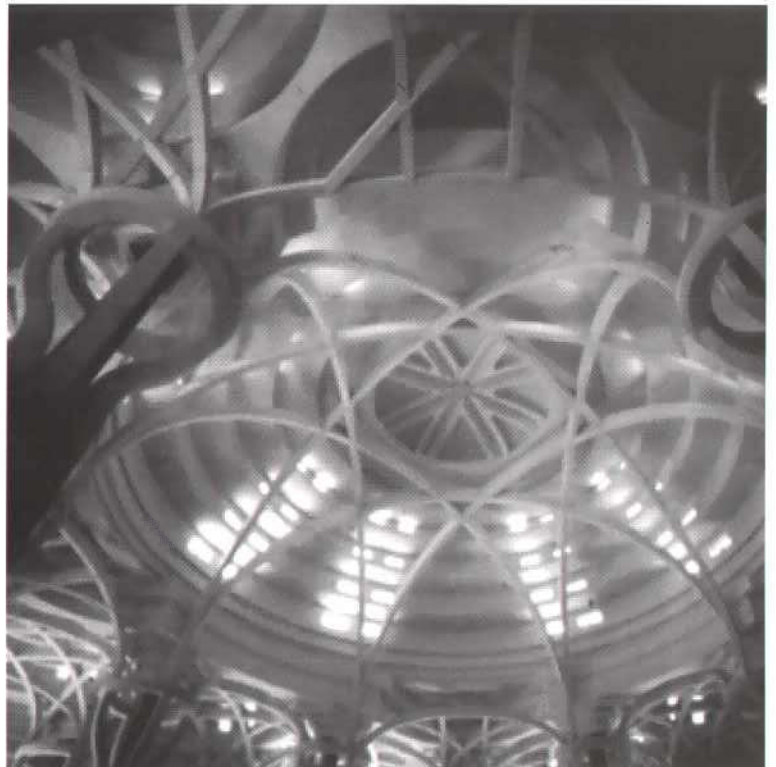
The Grand Mosque in Sarawak was designed with Sami Mousawi. The dome is made from a large laminated-timber, lattice grid-shell and is supported by a complex precast-concrete structure.
