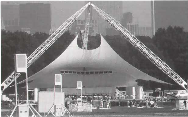
Carlos Moseley Music Pavilion Arch+Engr: FTL-Happold Date: 1989-91
