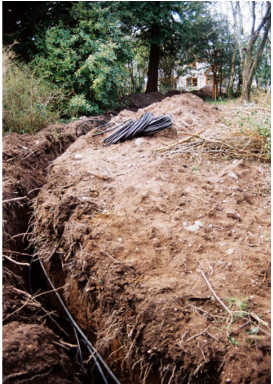
View of trench with slinky installed
