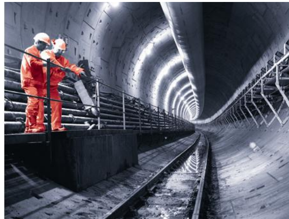
Image 6: Typical twin-bore tunnel 10
