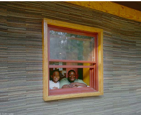
Innovative tectonic reuse of material here provides a home for the poor. Cardboard or stacked carpet tiles provide infill, while reused car windscreens act as cladding.
