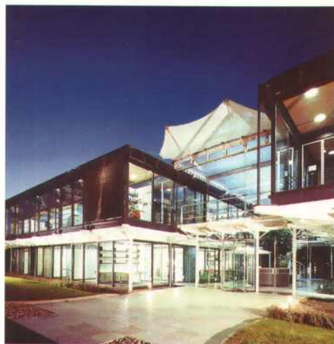
ETFE FOIL CUSHIONS: THE ROOF OF THE SECOND SCHLUMBERGER BUILDING, CAMBRIDGE, UK
