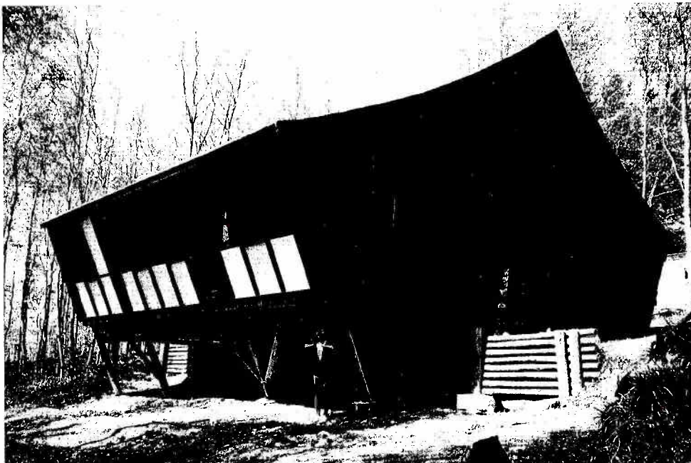
Fig 5.2 a) External elevation of completed prototype house
