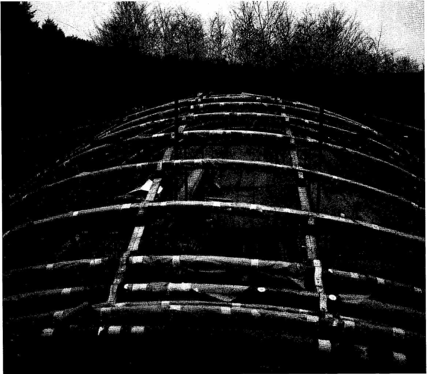
Fig 5.14 Construction of crown arch members
