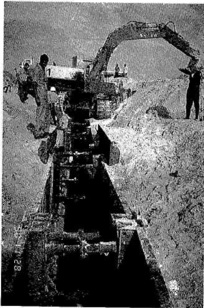
Fig 4.5 Ground work under way again on site
