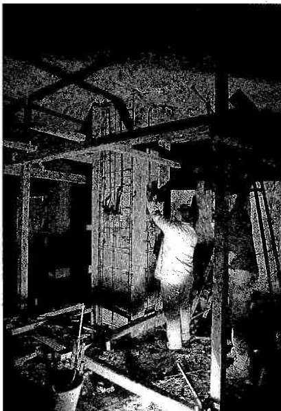
Fig 6.7 a Column being prepared for guniting
