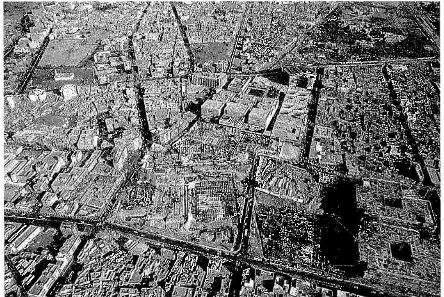
Fig 2.2 City centre during early construction of Kasr Al Hokm development
