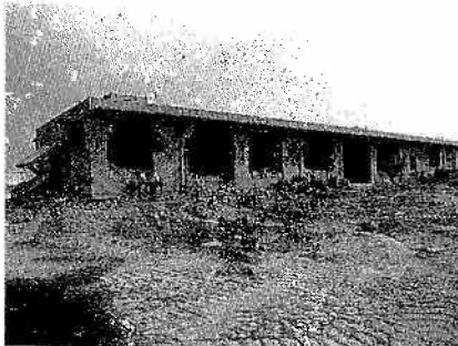
Fig 7.10 Destruction by tracked vehicle in MOD complex
