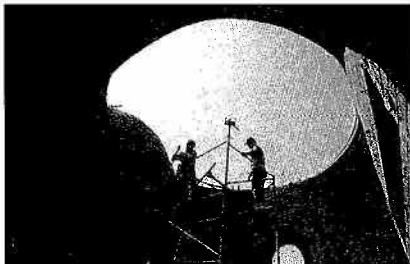
Fig 5.8 Typical construction without forms of larger dome
