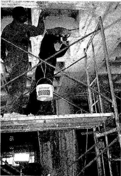
Fig 7.18 Resin injection of cracks in fire damaged concrete.
