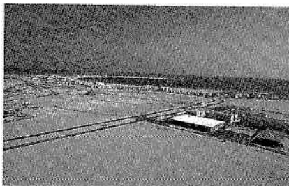
Fig 4.7 Phase 1, from microwave tower
