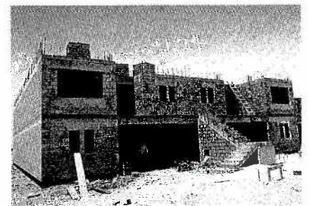
Fig 4.3 Structures following halt on work in December 1989
