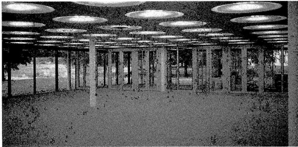
Fig 4.2 Coffier lighting and full height glazing on ground floor
