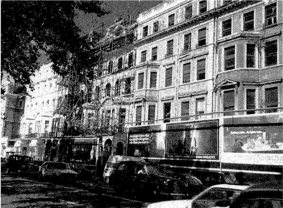
Fig 7.1 Cromwell Road facade, prior to refurbishment
