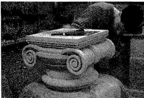
Fig 7.11 Stonework repair in stonemason's workshop
