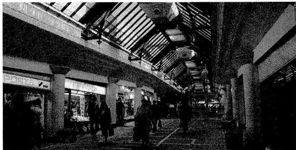
Fig 2.10 New glazed roof of refurbished Swan Walk shopping mall
