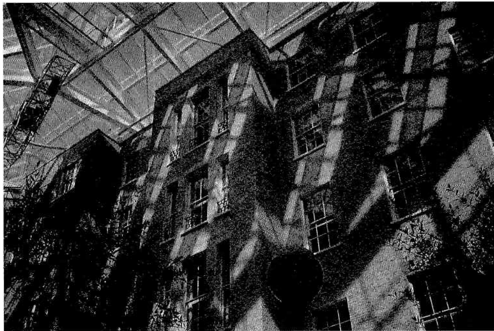
Fig 5.2 Inside the completed atrium courtyard
