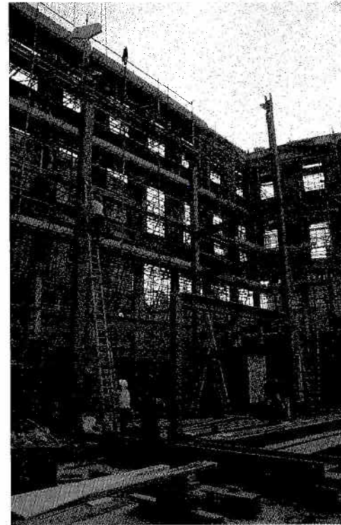
Fig 7.4 Shored facade standing alone above excavated basement
