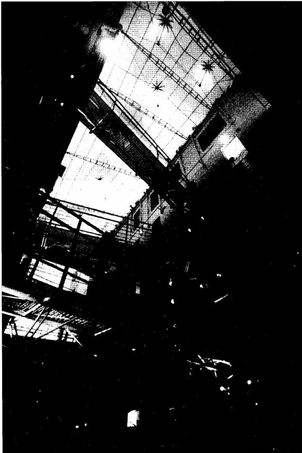
Fig 2.9 Multilevel linking walkways within atrium
