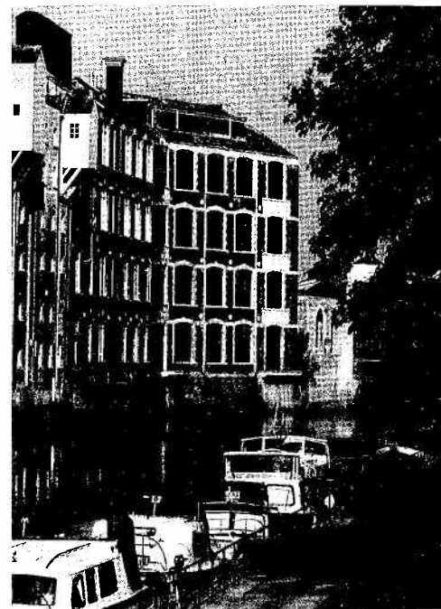
Fig 4.8 Refurbished river elevation
