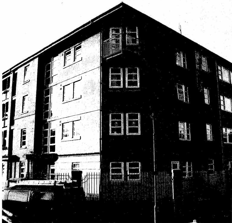
Fig 6.10 View of new NE corner block
